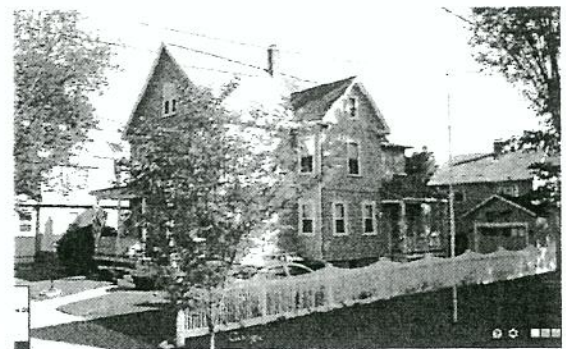
This is 24 Washburn Street in Newton, photographed when it was Bubba's childhood home in the early 1900s, and today. It has hardly changed in 100 years.
