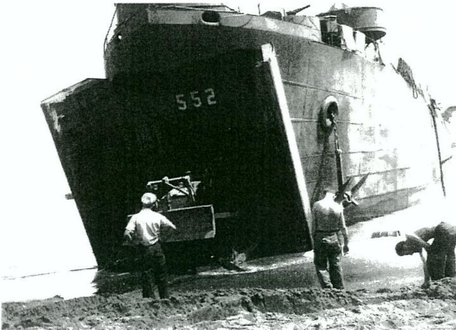
This is a photo of Dad's ship in action. Because of its usefulness, a bulldozer was the last thing loaded and the first thing off an LST. It filled holes and carved a road for the rest of the vehicles. It also towed or any tanks, trucks or jeeps which broke down or got stuck.
