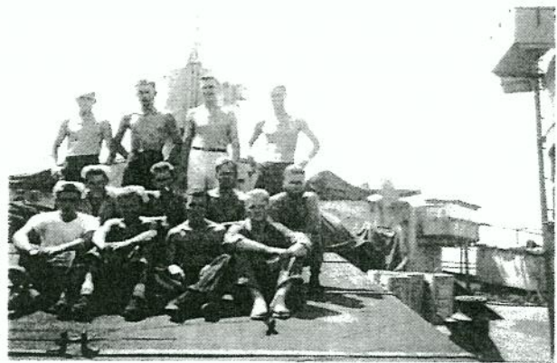
Some of LST 552's crew topside.
